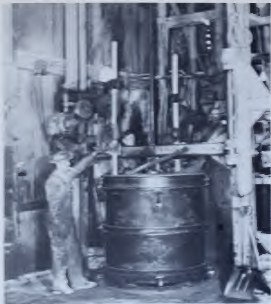
Figure 189—Equipment for manufacture of reinforced or unreinforced tamped concrete pipe up to about 54-inch diameter. PX-D-54073.
